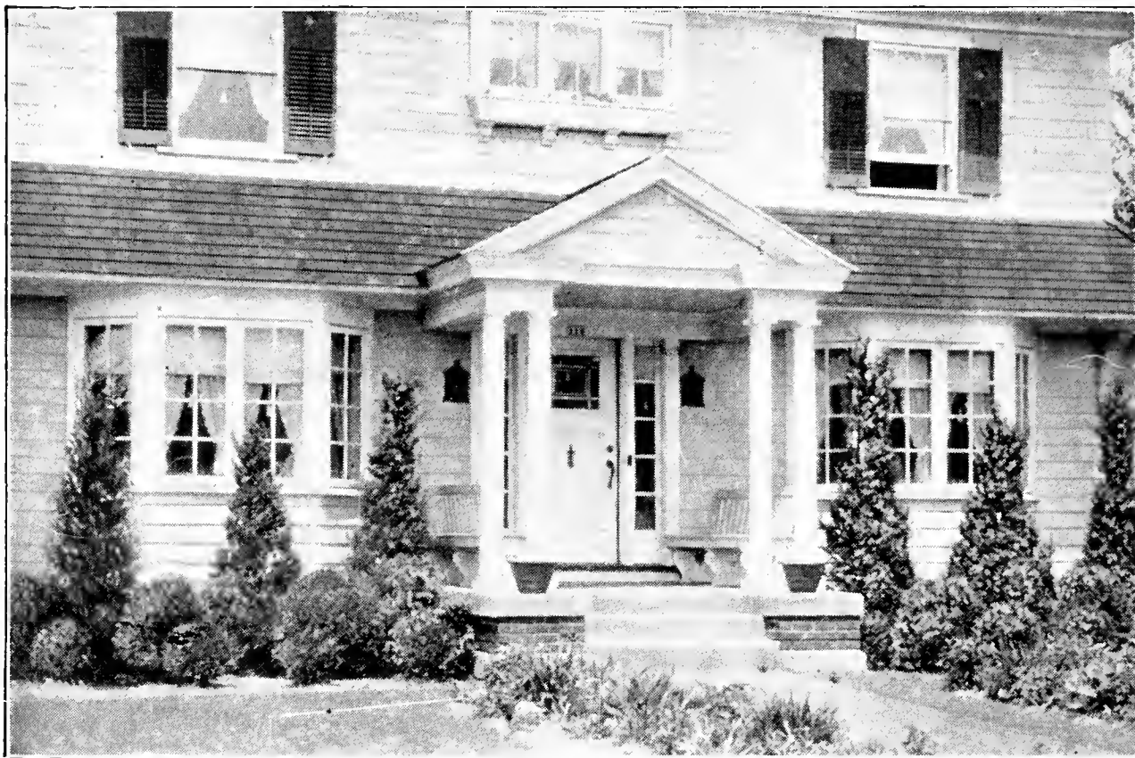
A Foundation Planting of Evergreens.
